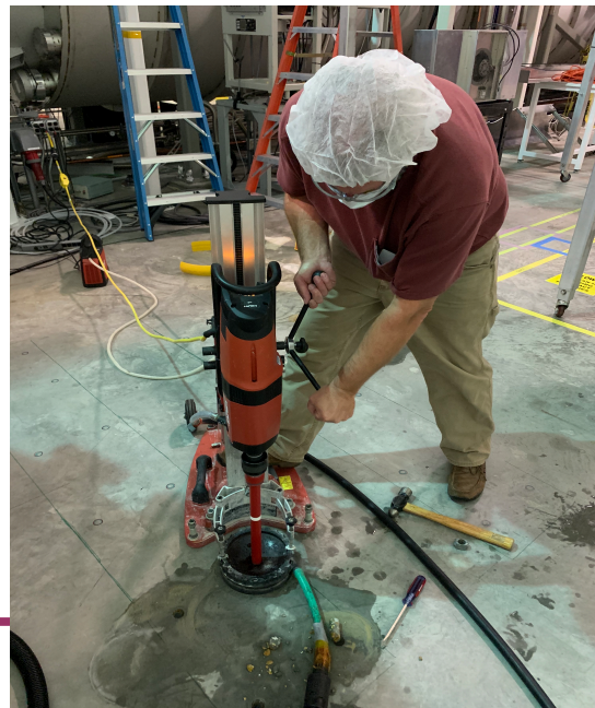
LHAM7 core drilling
