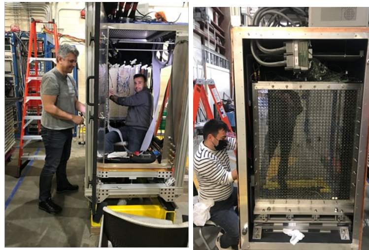
Mikta Imre and Carlos Domingues installing PMT/bases assemblies
